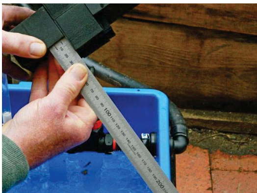
20 mm gap between the bottom of the float and the bottom of the slides
