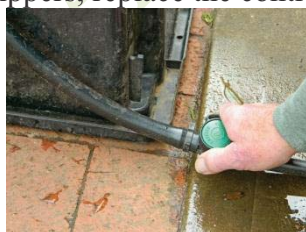
Open the main valve and the irrigation starts
