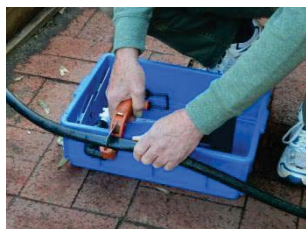
Cut the water supply pipe
